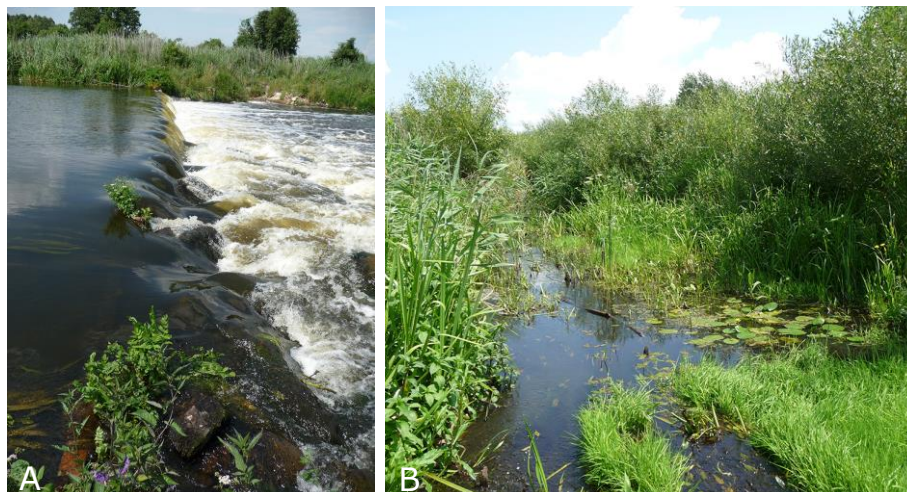
Figure 1.19 Upstream study reach: one of the submerged sills that is present a few hundred meters upstream of the restored reach (A) and a secondary channel with abundant aquatic vegetation (B).
