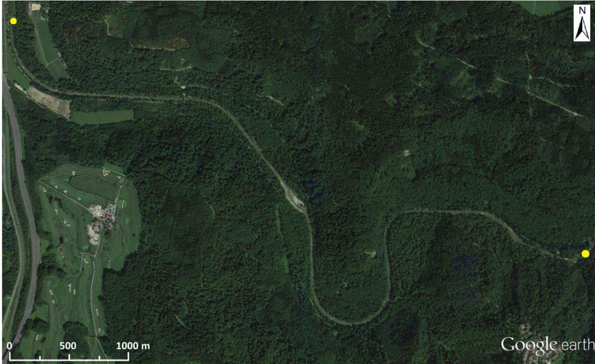
Figure 1.25 Aerial photo of the Töss River at the selected reach (Google earth, 2012).
