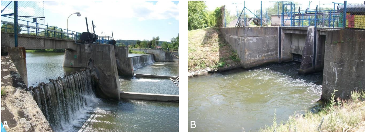
Figure 1.7 Diversion at the upstream limit of the degraded reach.
