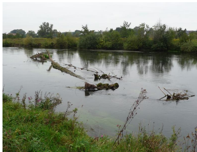
Figure 1.15 Upstream restored reach: one of the trunks that were fixed in the channel and on the banks, to enhance microhabitat diversity.
